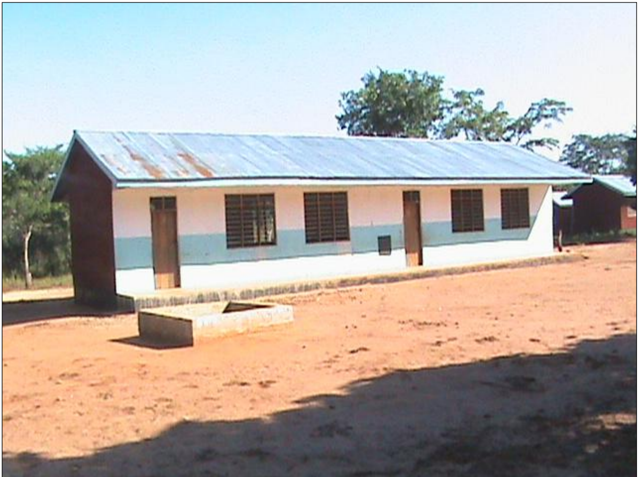
FIGURE 7: A TWO CLASSROOM-PRIMARY SCHOOL CONSTRUCTED IN LIWITI VILLAGE
