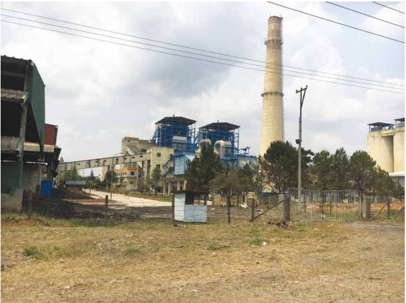
Tigyit Thermal Power Plant, which has been shut since 2014, will be run for a year on a test-basis
