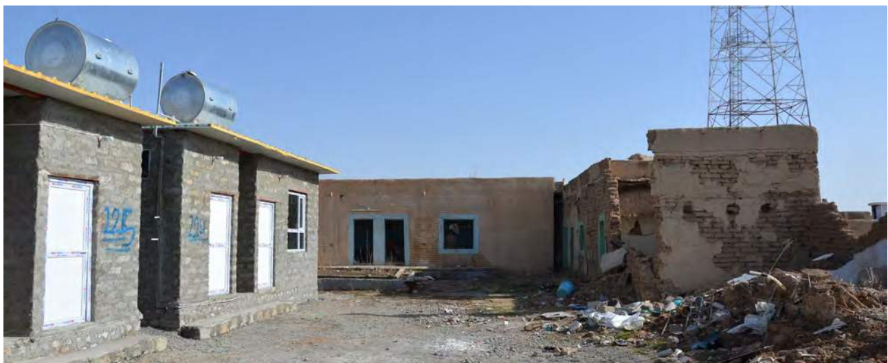
Rehabilitated housing units in Hardan, Sinuni-sub district, Sinjar, Iraq. Photo: UN-Habitat
